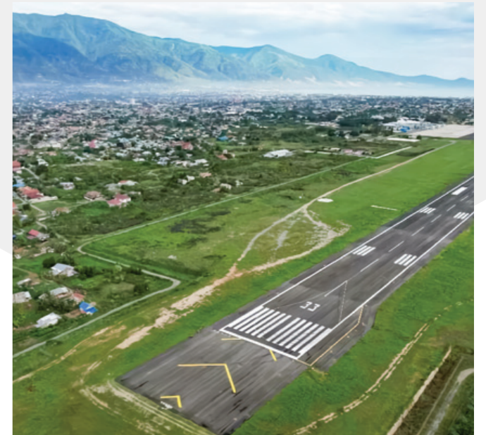
Runway Bandara Mutiara Palu
